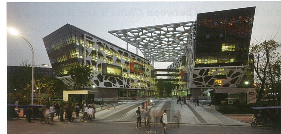
HASSELL's most talked about Chinese project, the Alibaba headquarters in Hangzhou.
