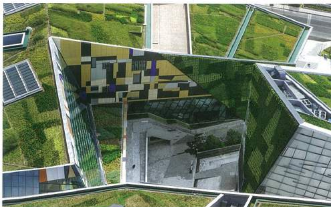
studio505's Phoenix Valley in Wujin showing the project's central valley and parts of its green roofs and facades.
