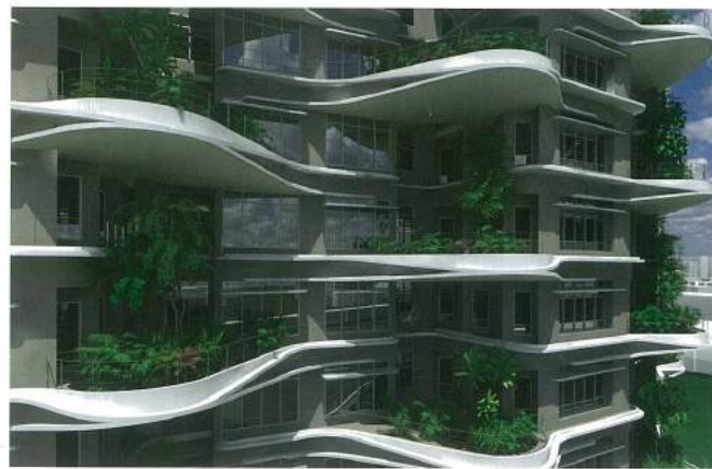
studio505's Ng Teng Fong General Hospital. External close up view of multi-bed, naturally ventilated, subsidised ward tower with external planter/gardens. (Courtesy: studio505 in collaboration with CPG, Singapore and HOK, USA)
