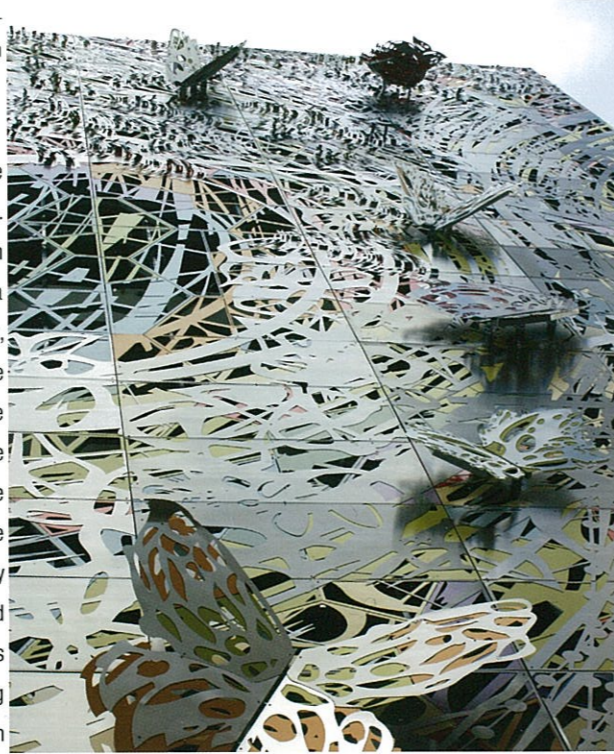
The butterfly element is used for the facade design
