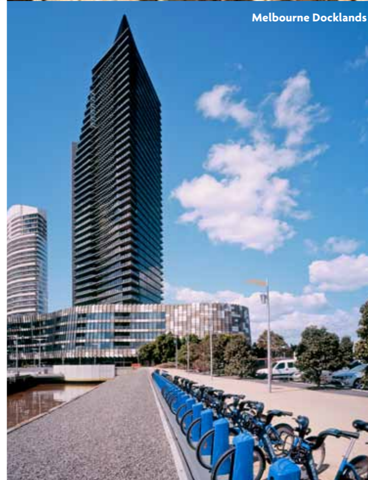
MELBOURNE DOCKLANDS PHOTOGRAPHY: GETTY IMAGES; PIXEL BUILDING: BEN HOSKING; EAGLE STREET: GPT GROUP
