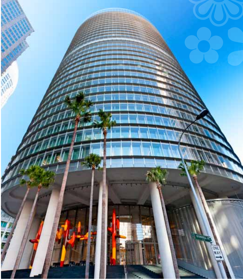
So sustainable: 1 Bligh Street, Sydney, features a double-skin glass facade and naturally ventilated central atrium
