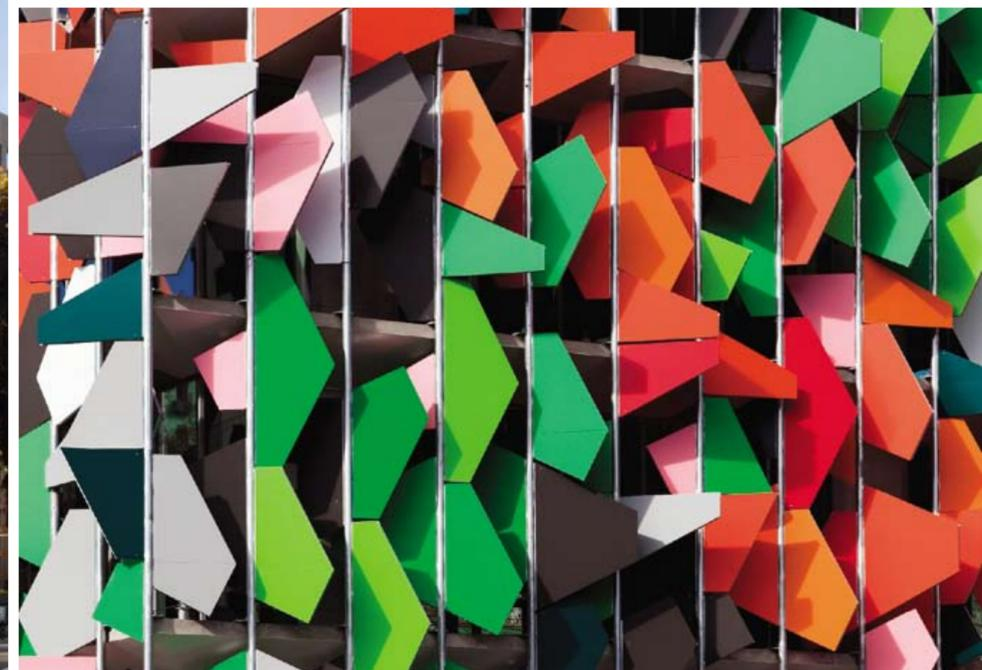
The Pixel Building has also been designed to provide 100 per cent daylight penetration into the office space, whilst allowing screen based technologies to be deployed without the need for blinds on windows. Extensive 3D CAD modelling was undertaken to maximise the performance of the external sun-shade system to promote daylight penetration.
