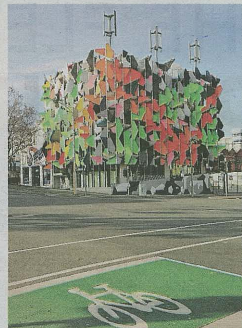
Multicoloured shade panels block solar heat, which helped the Pixel office building in Melbourne score six green stars.
