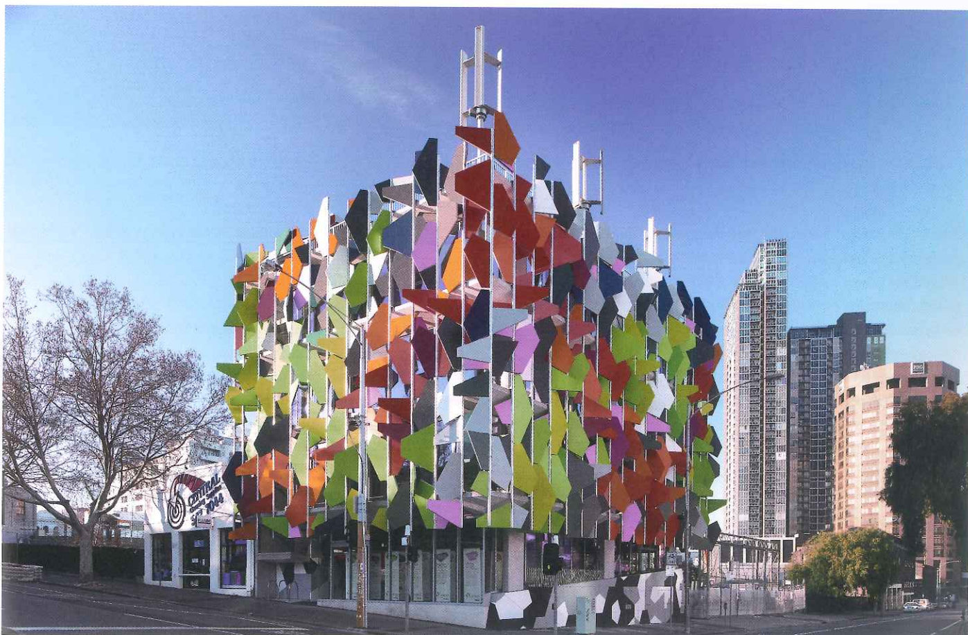
9.5 The multicolored fixed louvers on the Pixel building wrap around all four sides to create a “pixilated” sun shading system. Photo: Grocon.
